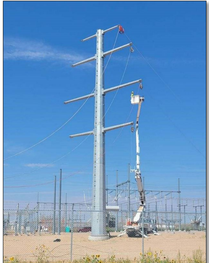
Crews prepare structure for the installation of insulators at the WAPA Ault Substation.
